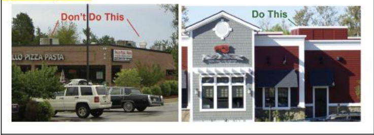
Figure <>: Rooftop Screening
