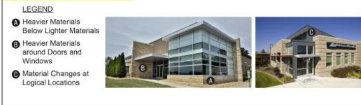
Figure <>: Commercial Building Materials
